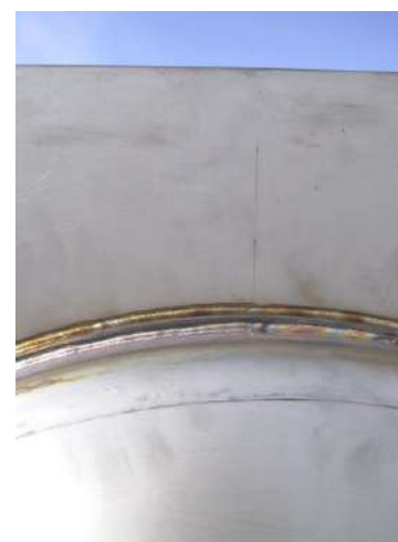
welding seam before using Antox
