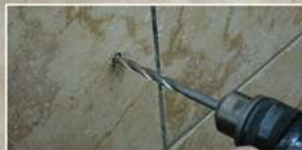
A hole is being produced in the substrate behind the tile with a suitable drill bit for the material being drilled
