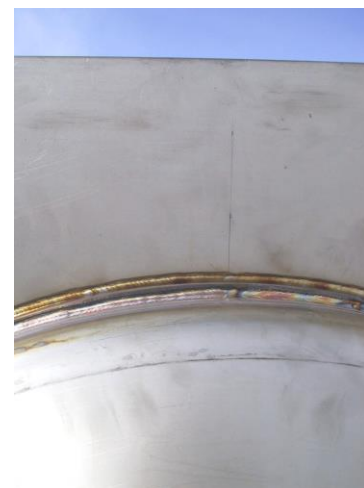
welding seam before using Antox
